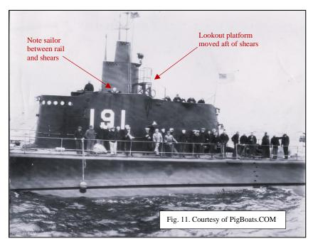
Figure 11 is Sculpin, taken during the Squalus salvage operation, June 1939. It is a good view of the conning tower fairwater. The portholes for the covered pilothouse are on the left, followed by the bridge, the periscope shears, a lookout platform, and the bulwark around the cigarette deck. Note that the lookout platform is aft of the shears, not alongside them as in previous boats. There is also a sailor leaning against the outboard of bulwark shears.
