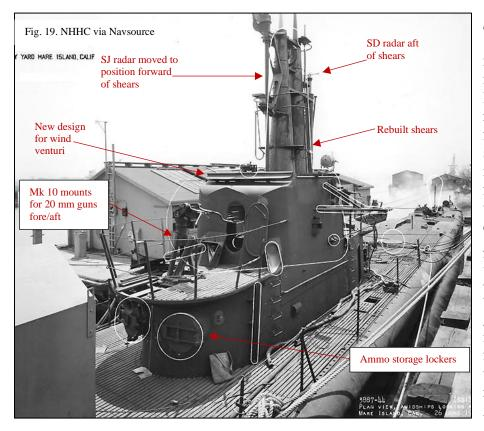
Seal, shown in Figure 19 in June 1944 has most of the late war modifications typical of later fleet boats. The SJ radar has been moved from its original starboard position and is now mounted directly forward of the shears with the SD radar mast directly aft. The 20 mm gun mounts are now the later tripod Mk 10 type, and an access door for the forward fairwater gun deck has been cut into the bridge fairwater. The bridge wind venturi has been rebuilt and repositioned. Ammunition storage
