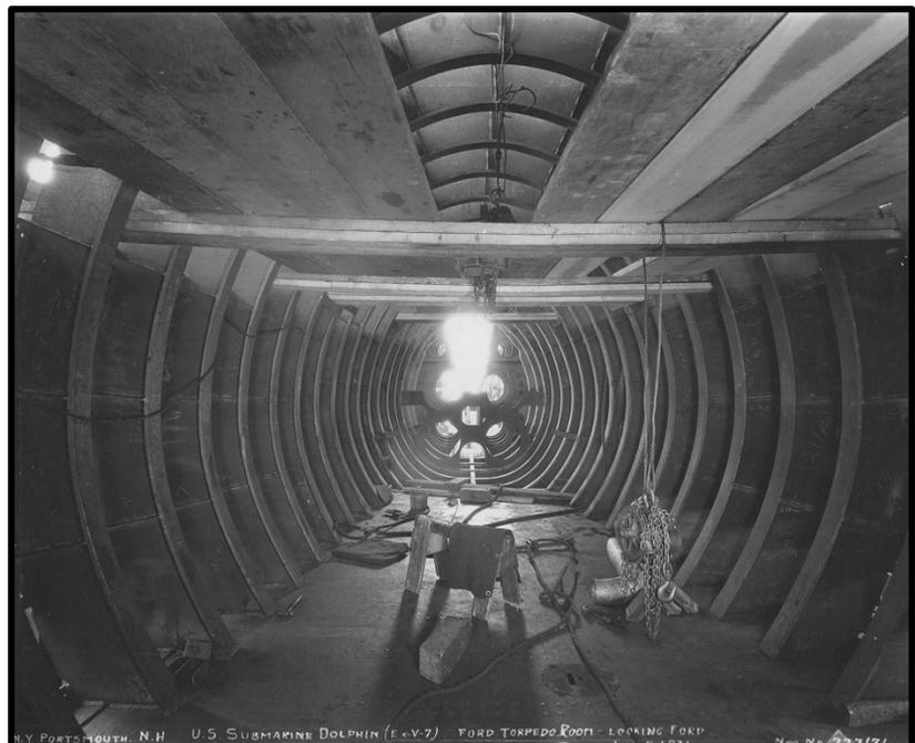
Figure 8. Dolphin forward torpedo room while under construction at Portsmouth, 1931. (NARA College Park photo courtesy of Tracey White and Navsource.com)
