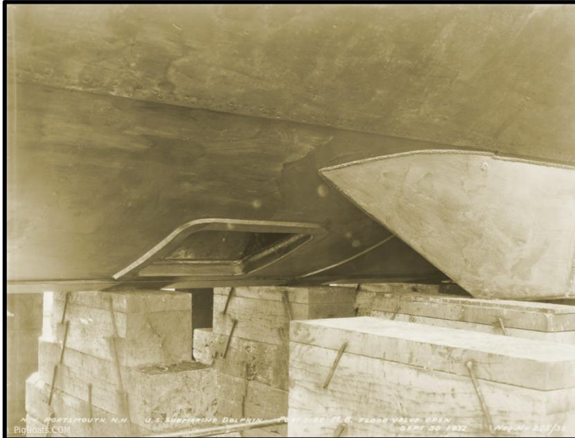
Figure 7. View of Dolphin's keel area, showing welded flood port flange and welded bilge keel. (NARA photo courtesy Roger Torgerson and PigBoats.COM)
