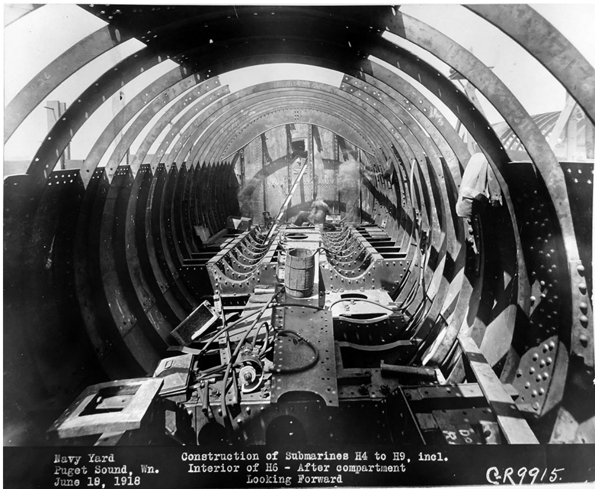
Figure 55. H-6 Engine Room.
