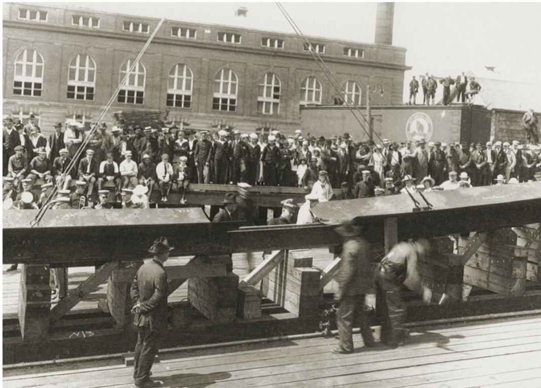
Figure 52. O-2 keel laying.
