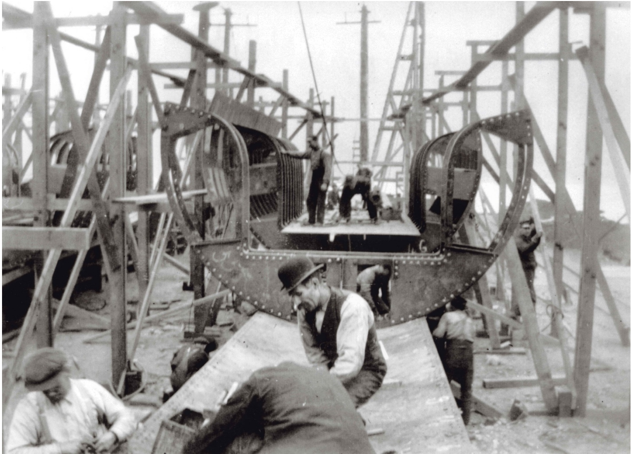
Figure 54. Framing in progress.
