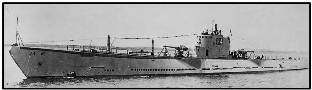
Figure 5. USS V-4 (SF-7) during sea trials off Provincetown, MA, June, 1928. This boat, not Cuttlefish, was the first submarine in the USN to incorporate welding in its construction. Three years after this photo was taken, she was renamed Argonaut. (USN photo via Pigboats.COM.)
