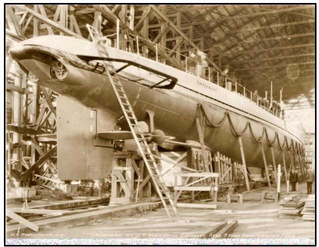
Figure 10. USS Cachalot (SS-170) on the ways at Portsmouth, 18 October 1933. While this picture is not detailed enough to verify the presence of welding, many of the seams on the outer hull appear to have been welded. (Rick Larson collection courtesy PigBoats.COM)
