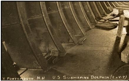
Figure 9. Closeup of Dolphin's forward torpedo room, clearly showing both welding and riveting. (NARA College Park photo courtesy Tracey White and Navsource.org
