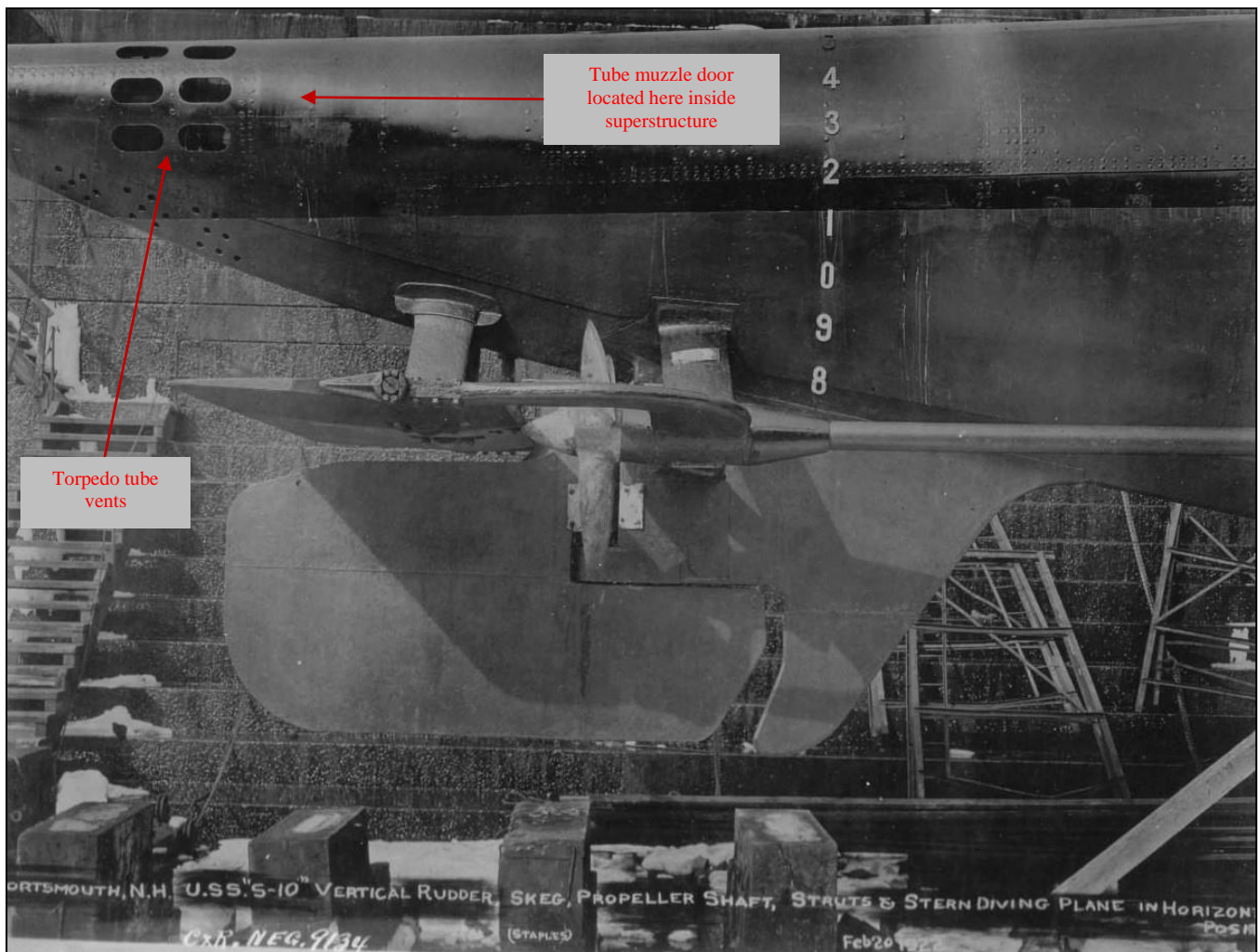
Fig. 9. Stern of S-10, 20 February 1922. NARA photo 19-N-9134 via Navsource.
